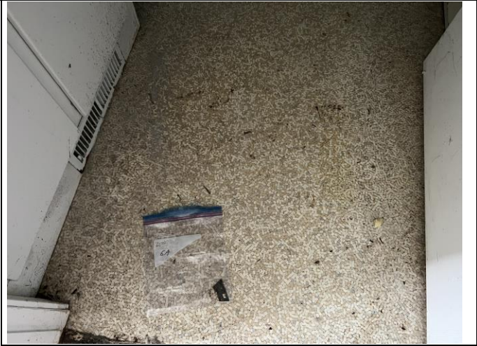
6. HM#6: Linoleum 1 & Mastic
