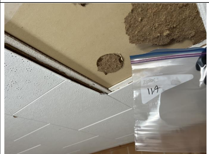
16. HM#11: Ceiling tile & mastic
